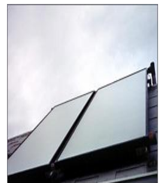
South facing solar water collecting plates
