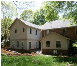
ADDITION WITH HARDI PLANK SIDING
